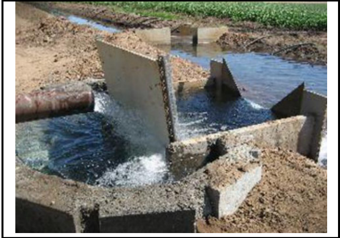
Example of an underflow baffle in a weir pool, in practice (Open Channel Flow Manufacturers, 2022)
